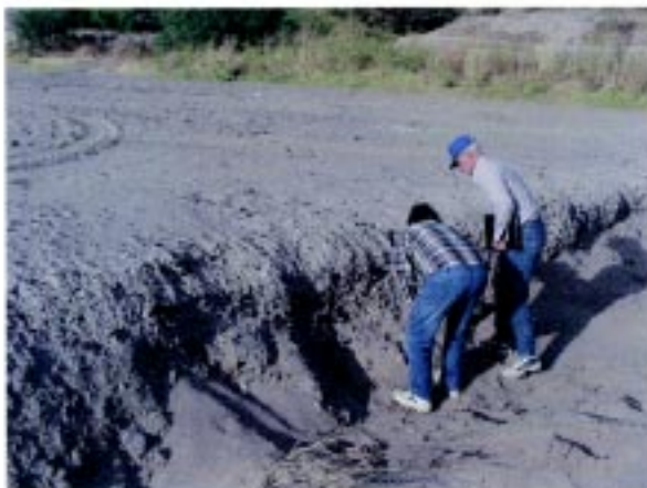
#3: Grade control structure S of Congress in the main channel
