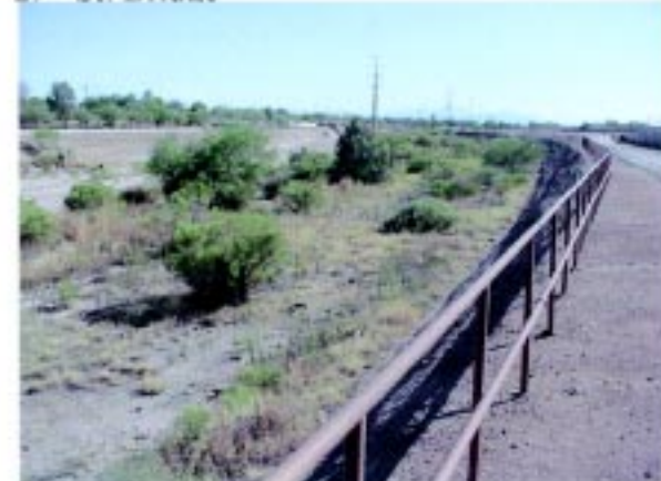
#12: View to S. of Santa Cruz channel 1/4 mile S of Ajo
