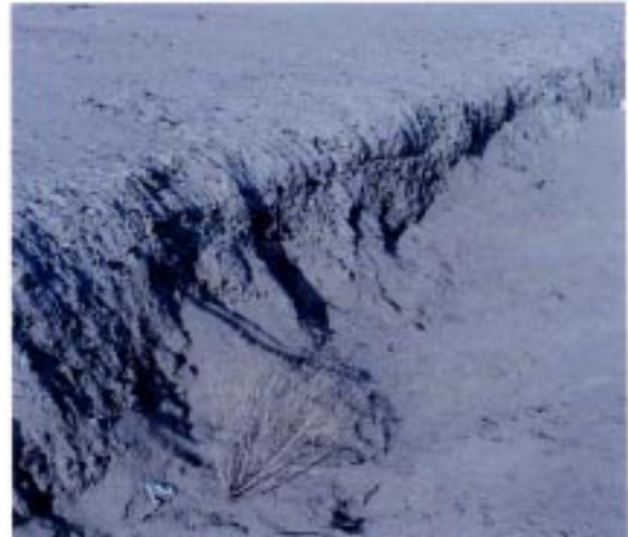
#2: Grade control structure S. of Congress in the main channel
