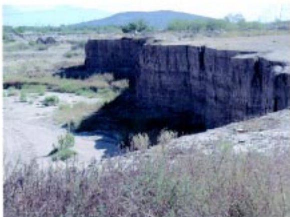
#25: Santa Cruz Riv. bank, south of Irvington (view to south) (closeup of previous photo)
