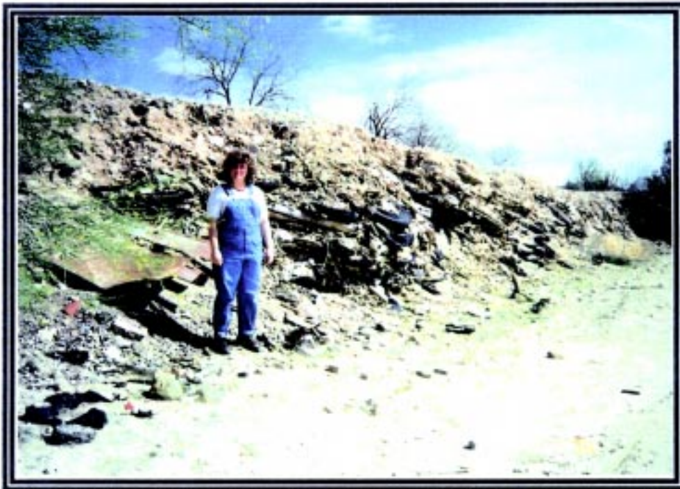
Photograph 5. Bank edge of Ryland Landfill at Site 22, view toward the southeast.
