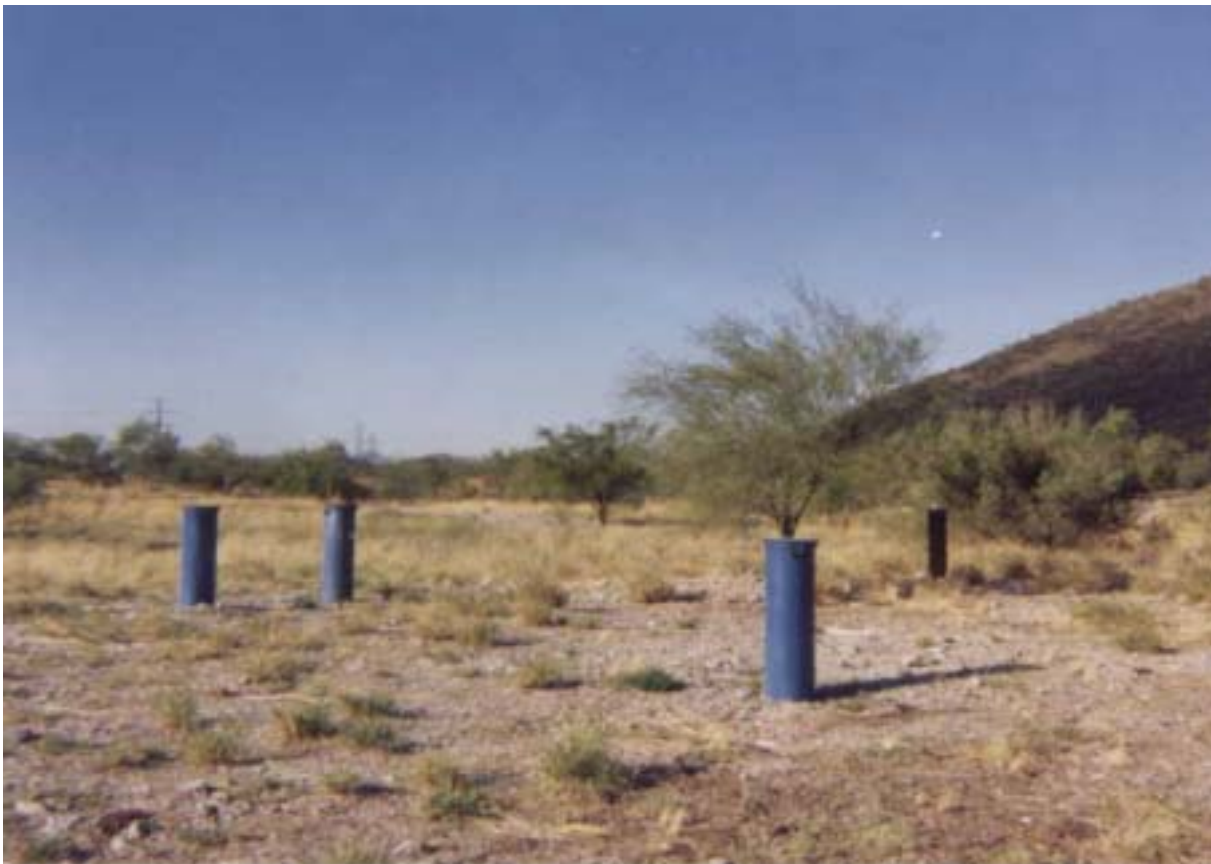
Photo 7: Water Monitoring wells near the Nearmont Landfill, south of Congress St., west of the Santa Cruz River
