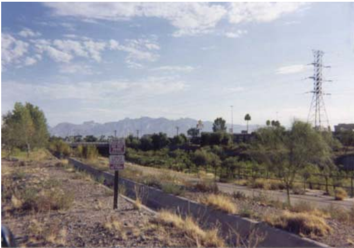
Photo 9: Irrigation ditch on top of riverbank, non-potable water for landscape irrigation; looking north towards Congress St. bridge
