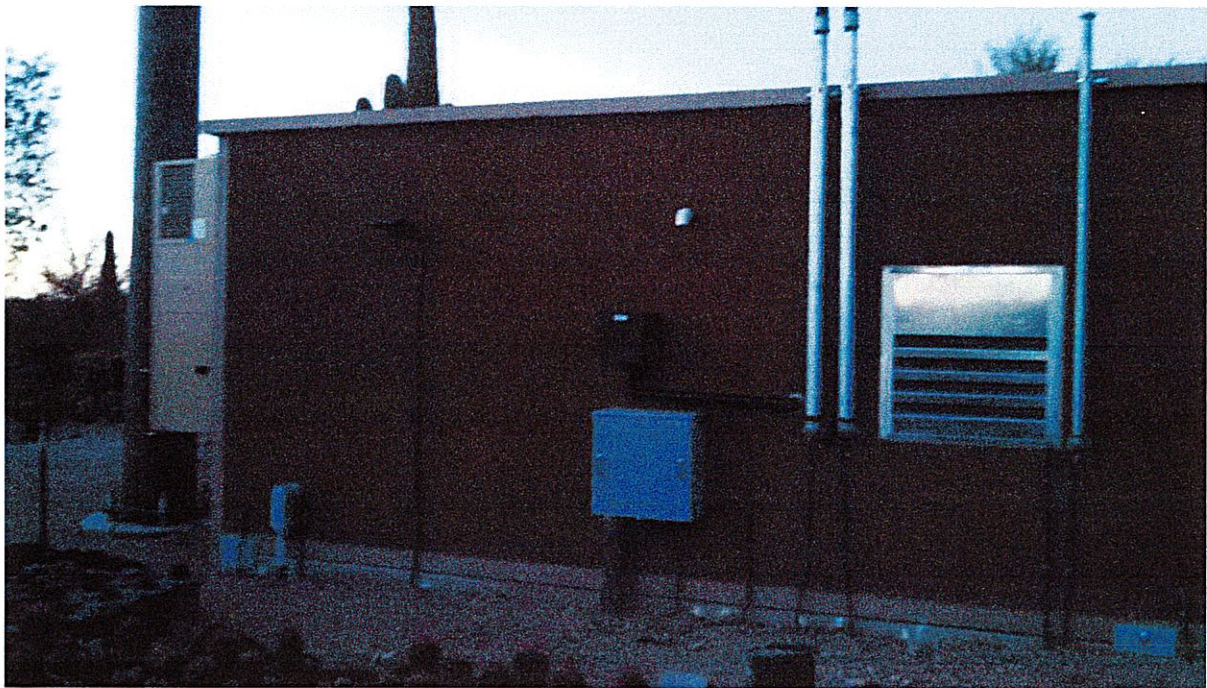
South face of building
