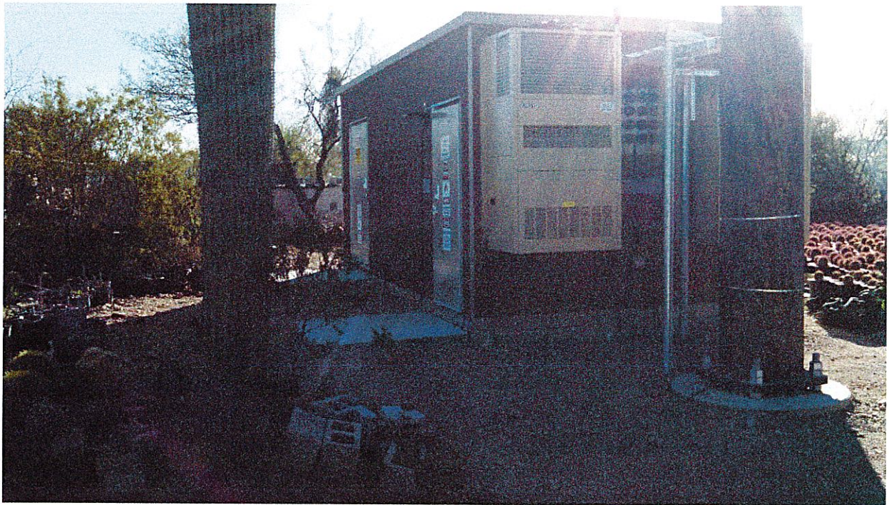
West face of building
