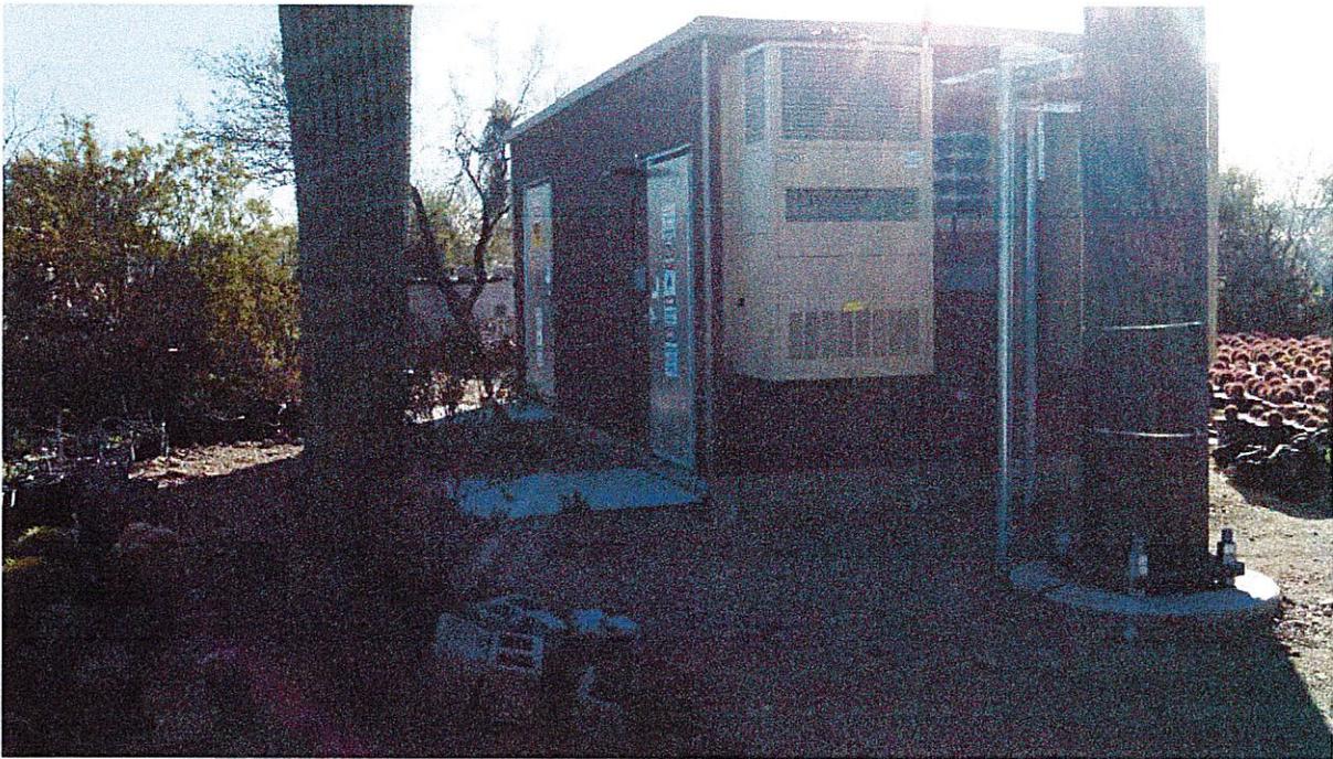
West face of building
