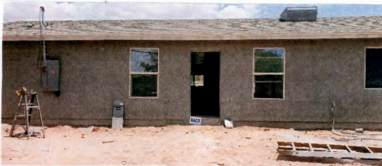
Back (looking N.) 2811 W. Quail Rd. 4/24/2011 (So. Side)
