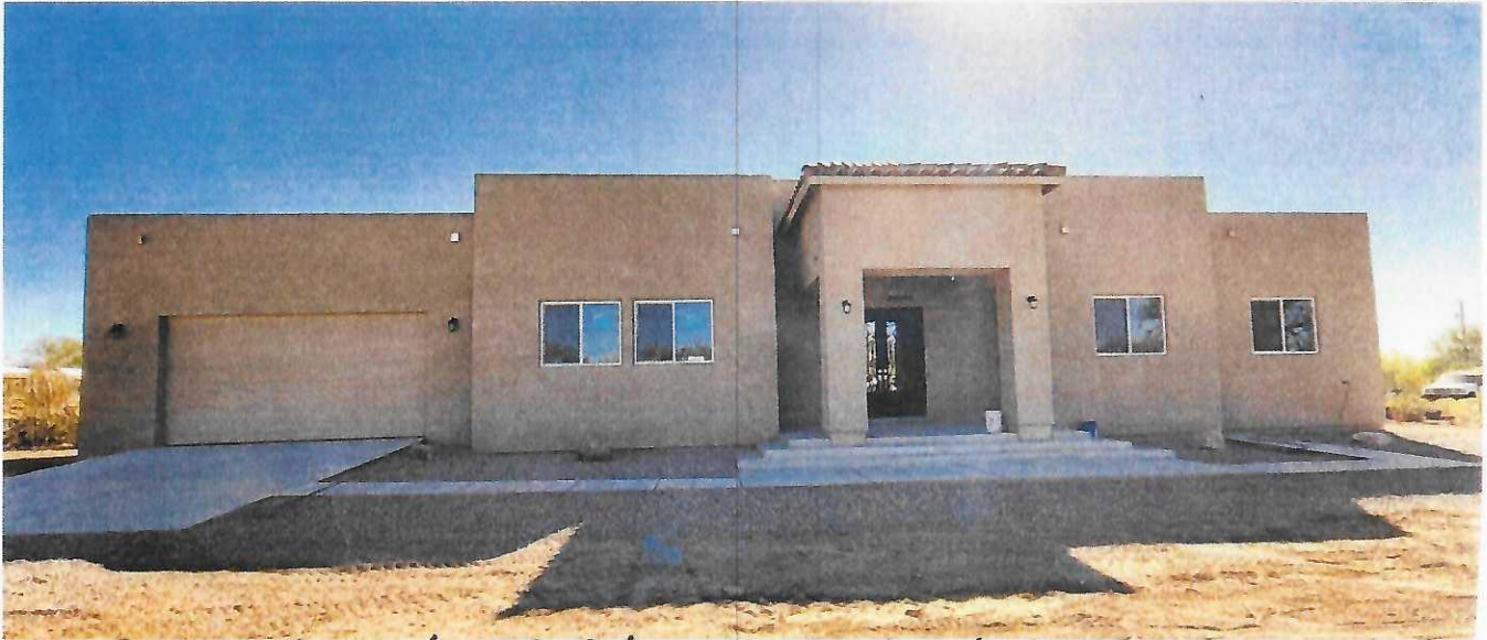
Front Side (W. Side Looking photo One East) 11/10/2023
