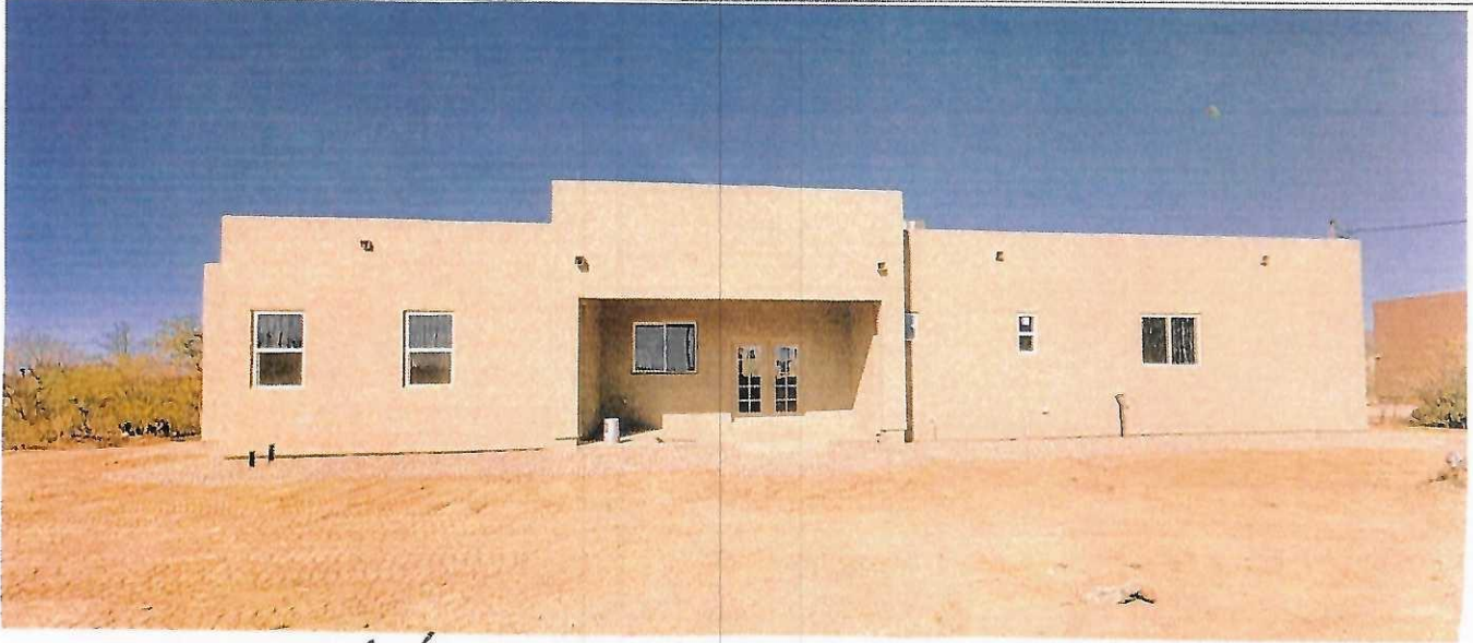
Back Side (E. Side looking W) Photo Three 11/10/2023
