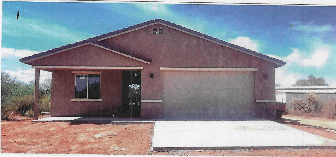
Front View (E. Side Looking W.) 10/9/2024 Photo One
