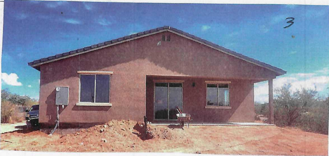
Back view (W. Side looking E.) 10/9/2024
