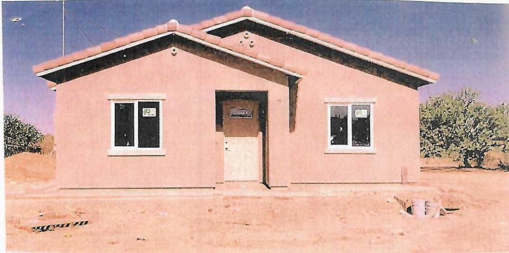
Front Side (E. Side looking West) 4/18/2024
