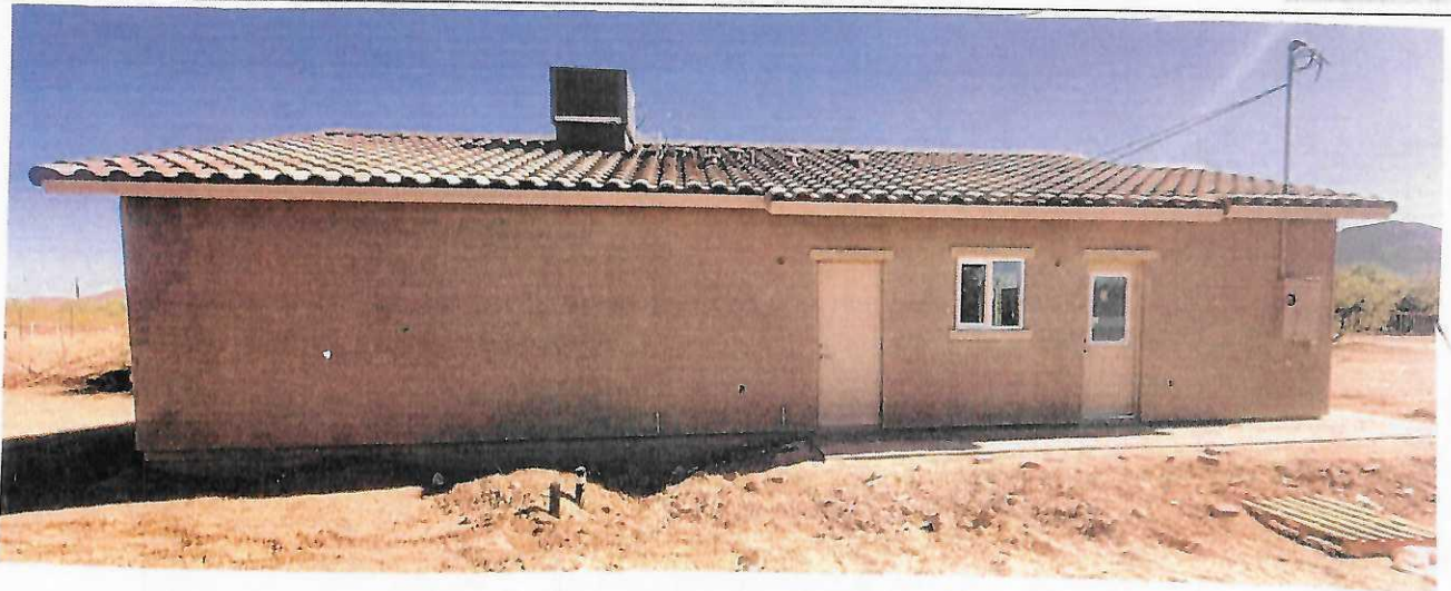
Left side (So. Side looking North) 6/18/2024
