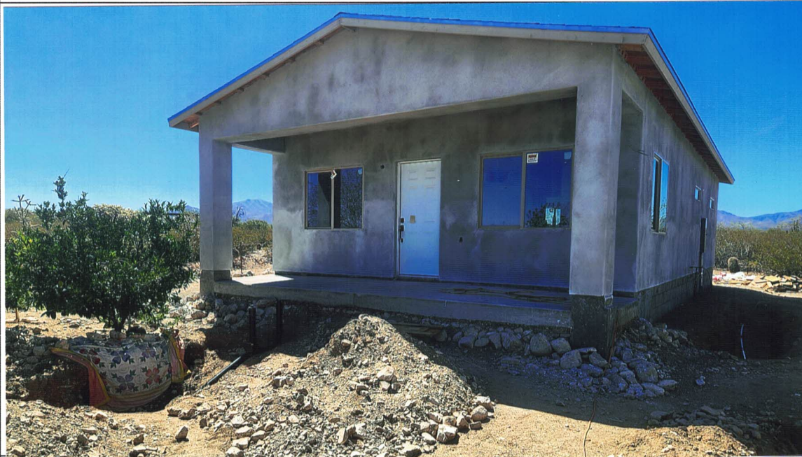
Photo One Caption: Front (North) photo date 5-7-25
