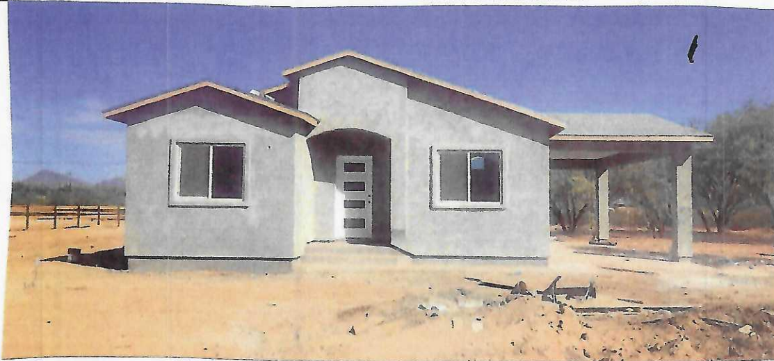
Front View (So. Side looking N.) 10/10/2024
