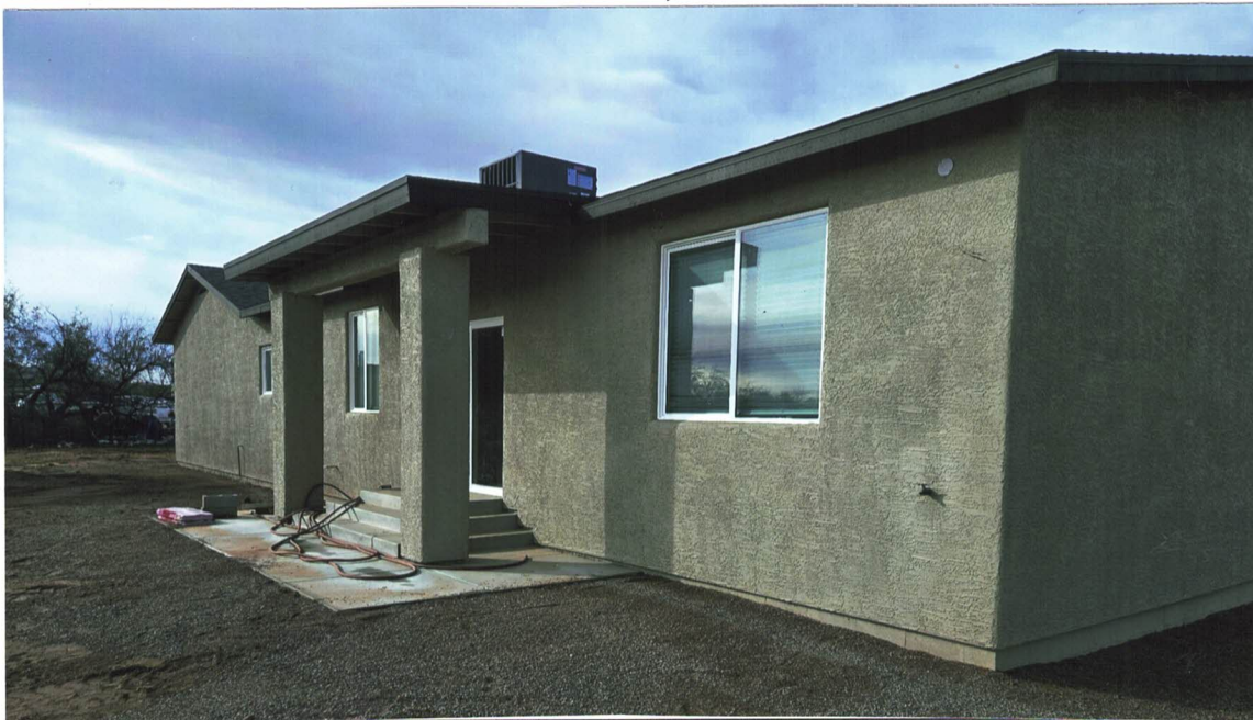
Photo Three Caption: Back (East) 1-26-25
