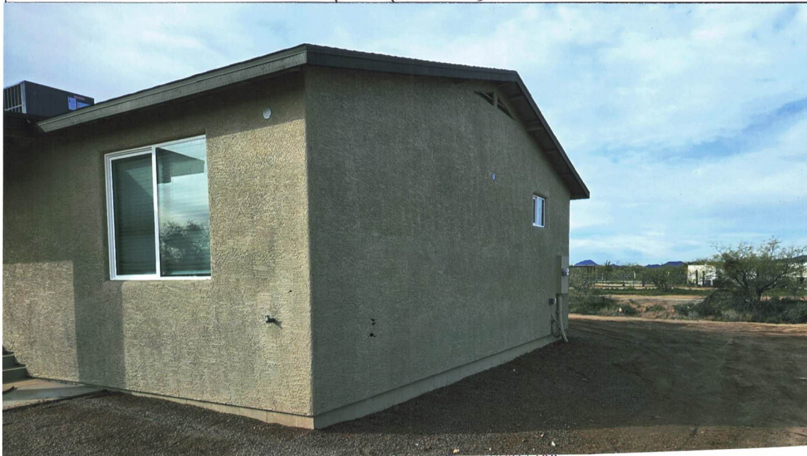
Photo Four Caption: Left Side (North) 1-26-25
