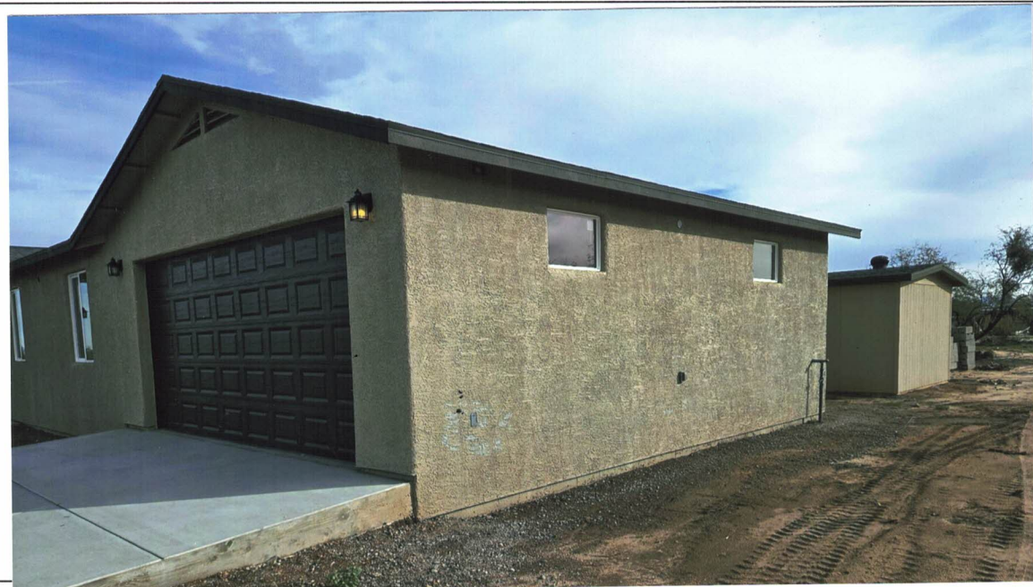
Photo Two Caption: Right Side (South) 1-26-25
