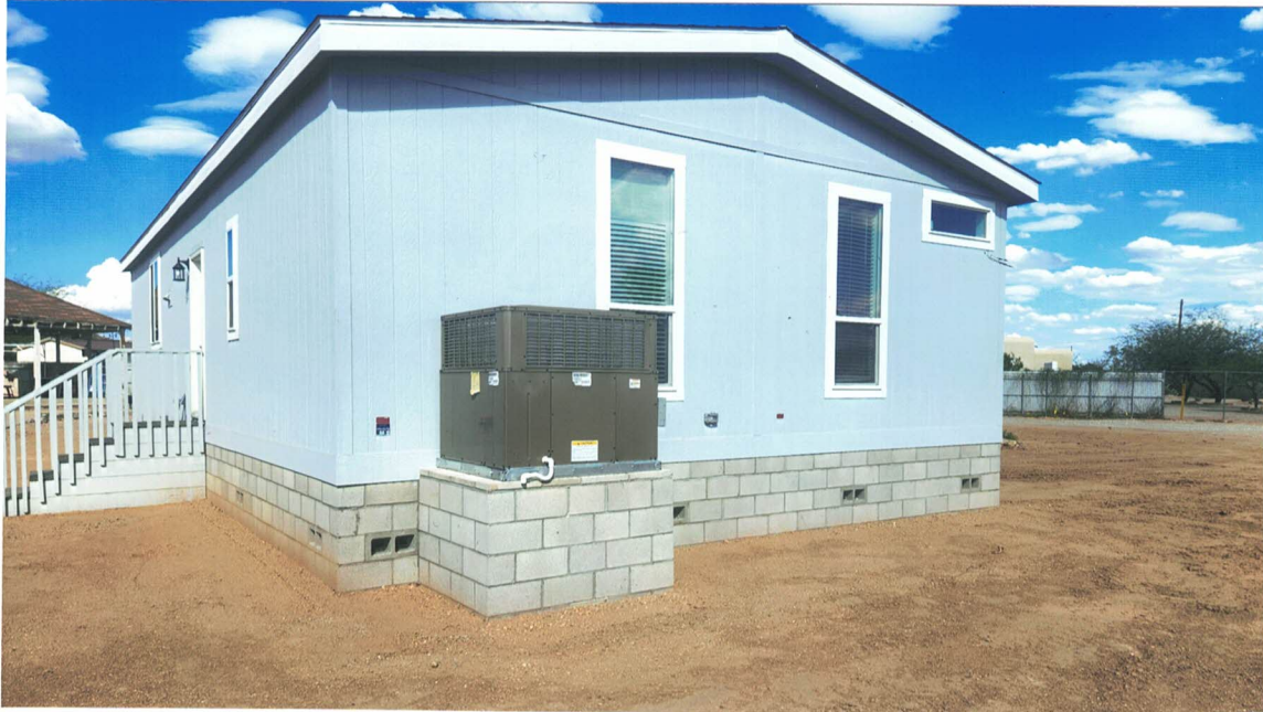
Photo Three Caption: Back (Southwest) 8/28/25
