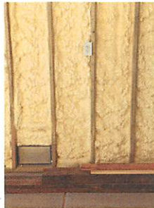
ELECTRICAL RECEPTICAL 4 FEET ABOVE FFE
