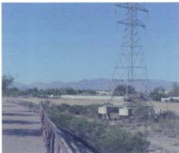
#22: Power pole base in Santa Cruz channel
