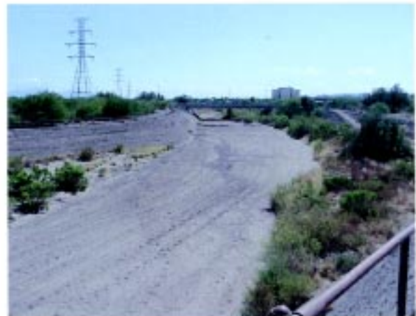
#8: View to S. of main channel (22 nd St Bridge in background)
