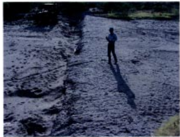
#4: Grade control structure S of Congress in the main channel
