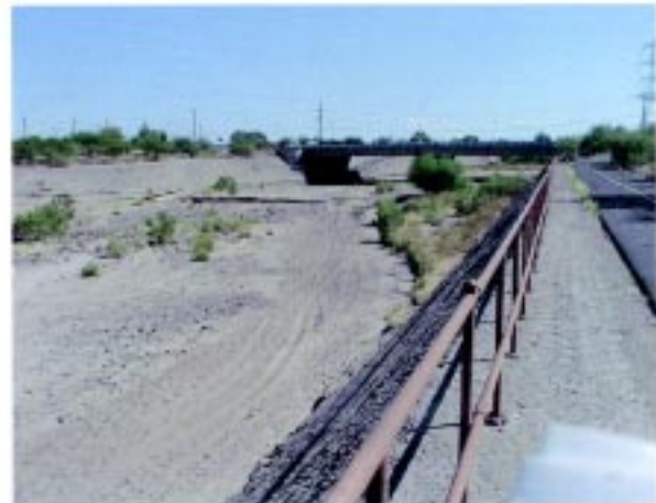
#10: View to S. of the main channel and the 29 th St. Bridge
