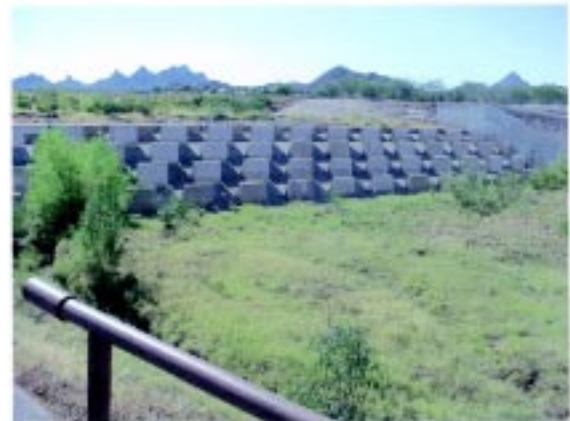
#27: Energy dissipation structure @ W. Branch just upstream of Santa Cruz River
