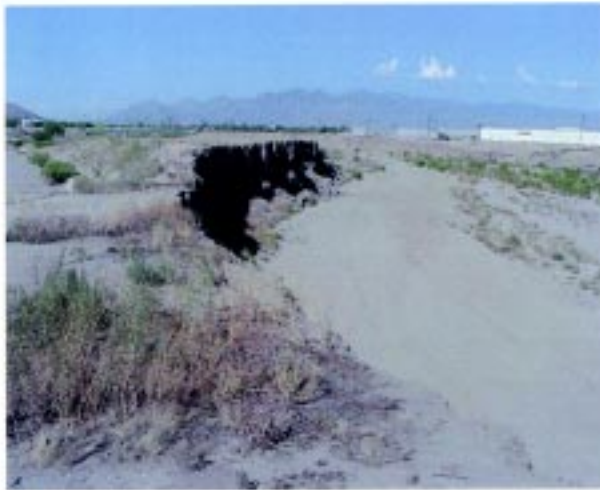
#23: Santa Cruz channel west bank, south of Irvington (view to north)
